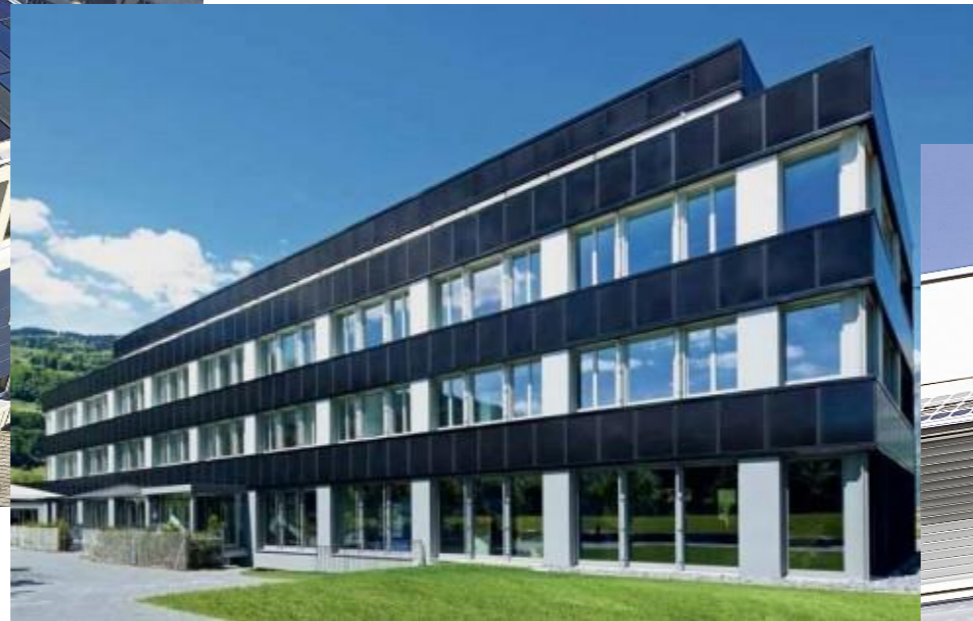
Flumroc HQ Flums PV Fassade PV Dach
