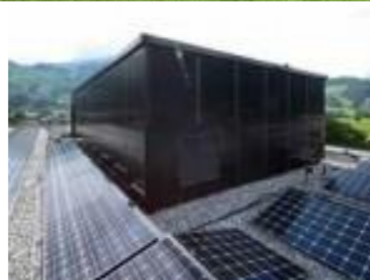
Flumroc HQ Flums PV Fassade PV Dach
