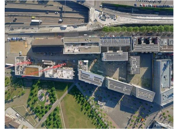
Erlenmatt Ost, Basel. © ADEV 200 Whg., 580 kW PV
